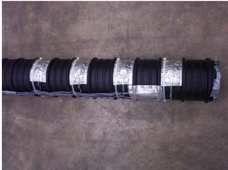
Figure 4.9 Completed Gage Installations on HD Polyethylene Duct
