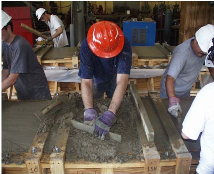
Figure 3.17 Concrete Finishing Operations
