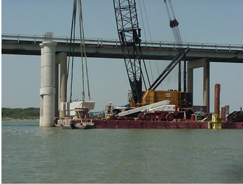
Figure 2.12 Bent Cap Placement Operation with Barge-mounted Crane
