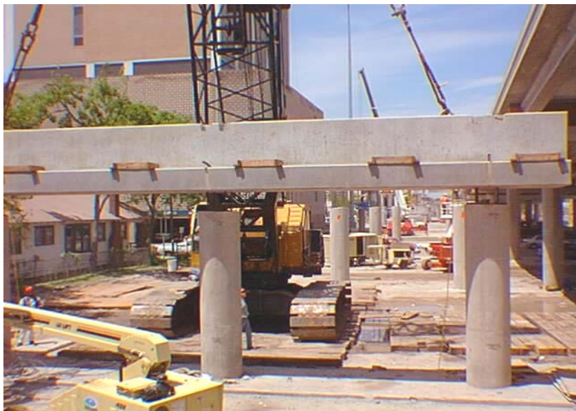
Figure 1.5 Pierce Elevated Project Precast Bent Caps
