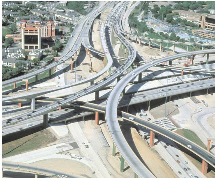
Figure 2.13 Aerial View of Dallas High Five Interchange Construction Site
