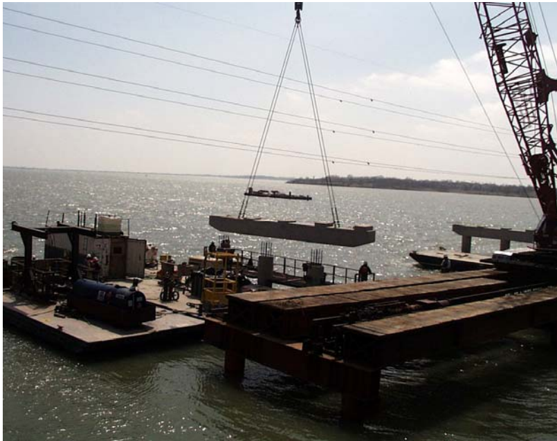
Figure 2.8 Bent Cap Placement Operations
