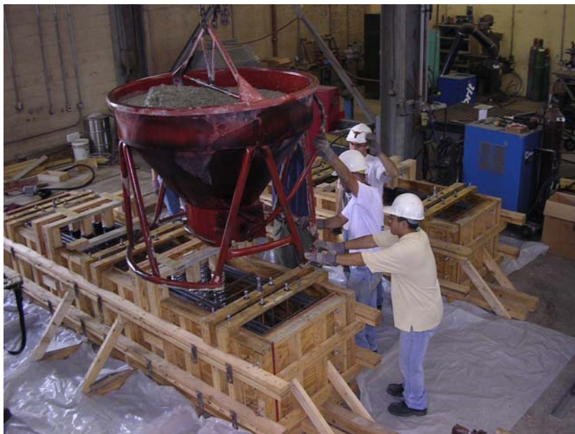
Figure 3.16 Specimen Casting with Aid of Crane-operated Hopper
