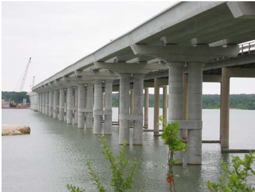
Figure 2.9 Construction of the Lake Belton Bridge
