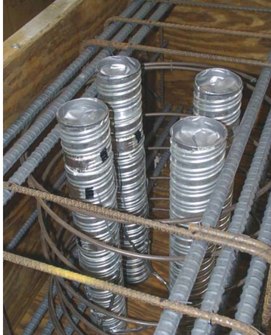
Figure 4.10 Completed Strain Gage Installations on Galvanized Steel Ducts
