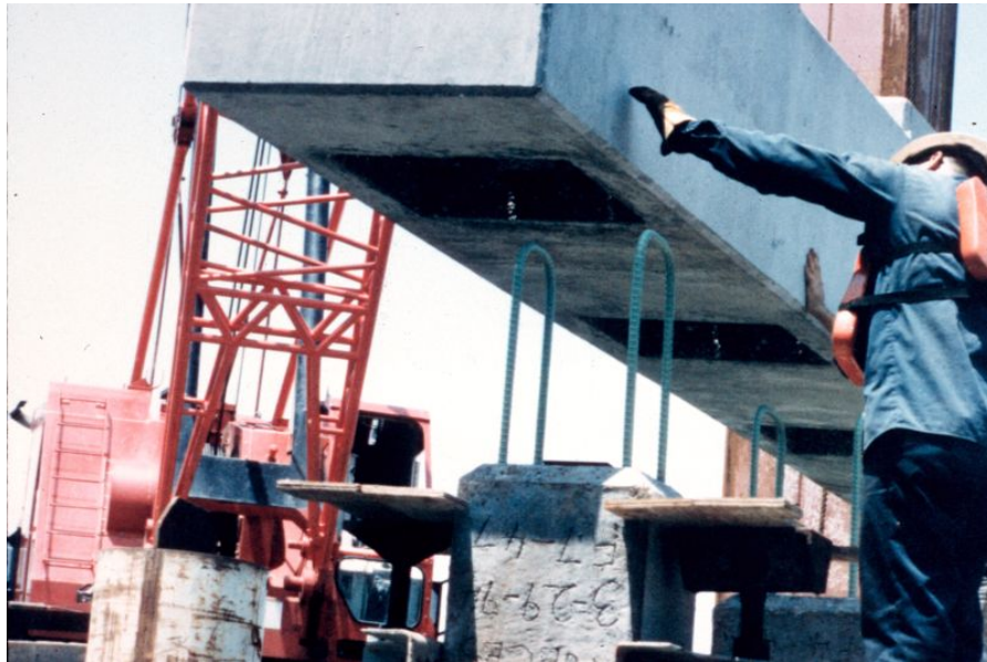
Figure 1.3 Red Fish Bay Project Precast Bent Caps
