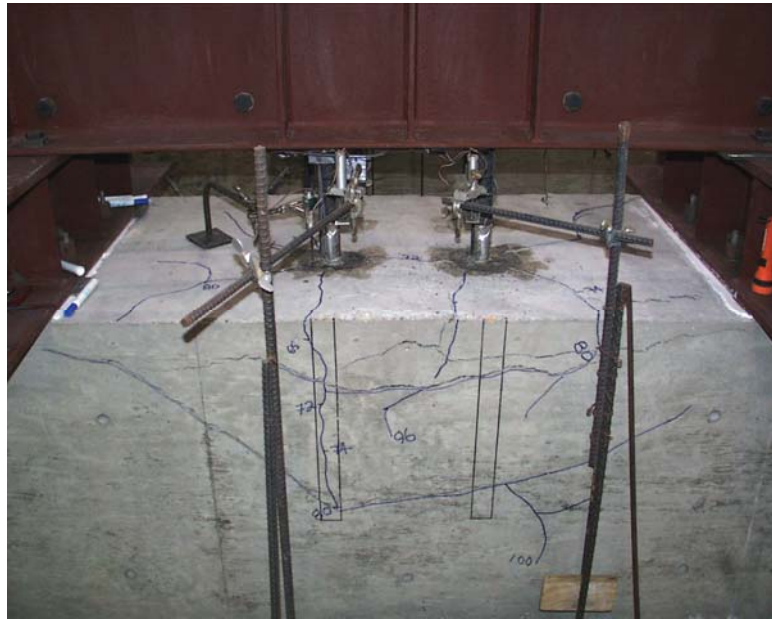
Figure 5.10 Double Connector Test with 2-D Duct Spacing (Test No. 23)
