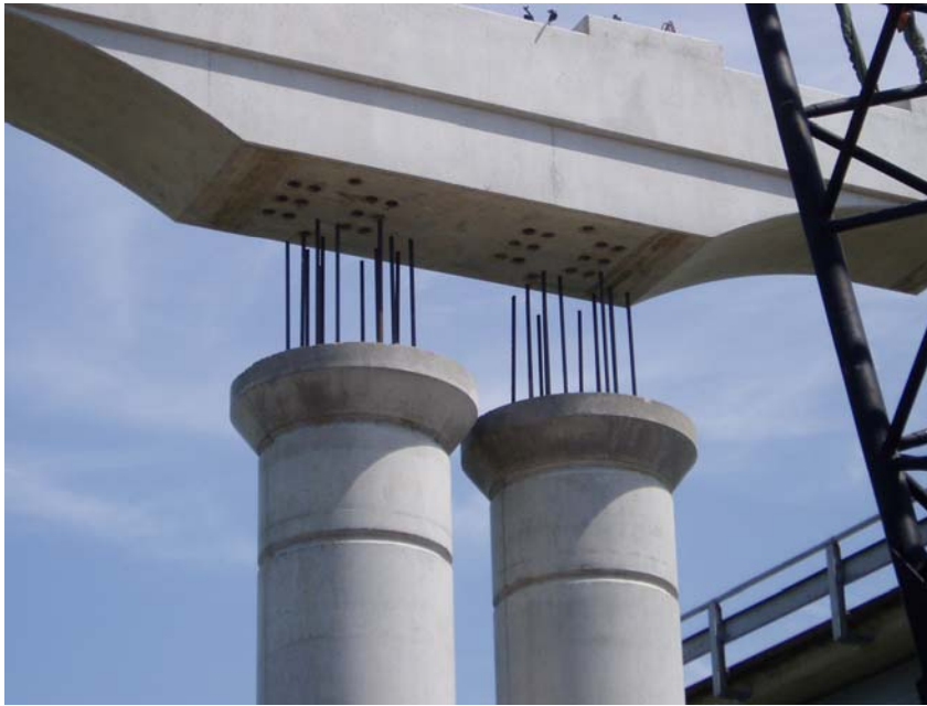
Figure 1.11 Lake Belton Bridge Project
