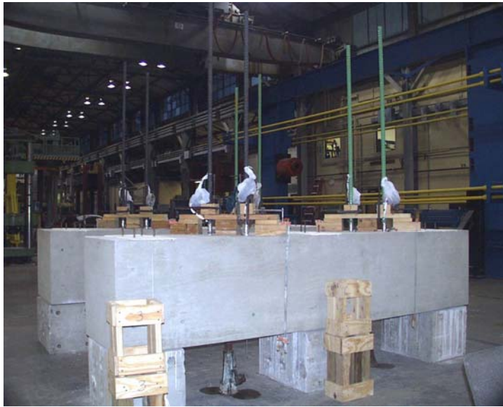
Figure 3.21 Positioning and Vertical Alignment of Connectors in Preparation for Grouting Procedures
