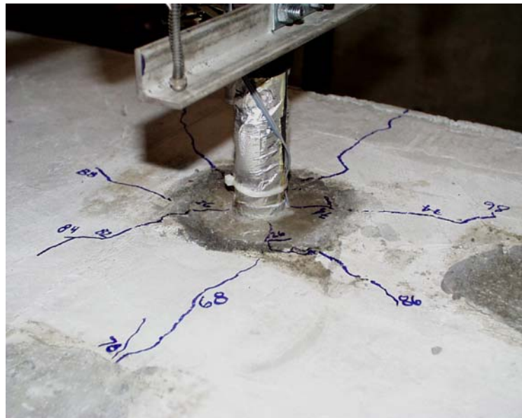
Figure 5.5 Widespread Splitting in Test No. 10
