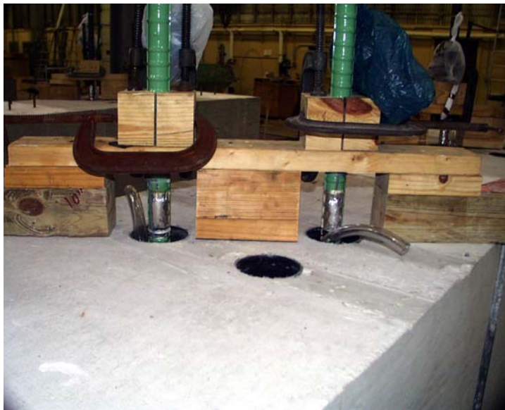
Figure 3.22 Formwork to Hold Connectors Aligned and in Place during Grouting
