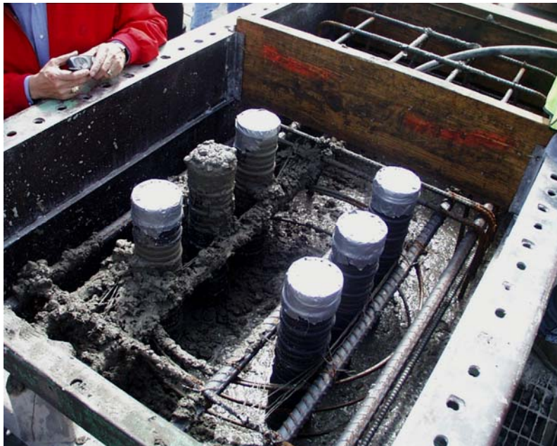
Figure 2.7 Bent Cap Connection Zone under Construction
