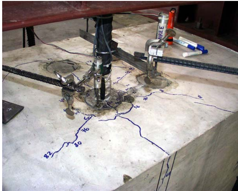
Figure 5.12 Test No. 9 at Failure Load
