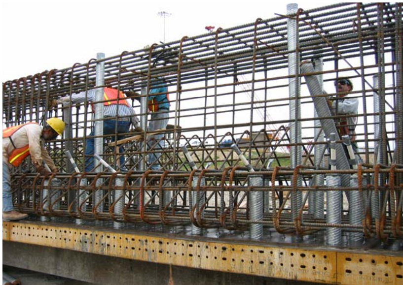
Figure 2.15 Placement of Bent Cap Reinforcement and Ducts
