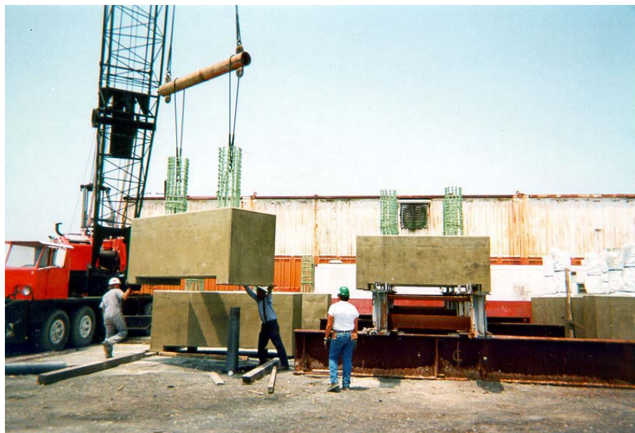
Figure 1.21 Beaufort and Morehead Railroad Trestle Bridge Bent Caps [1.23]
