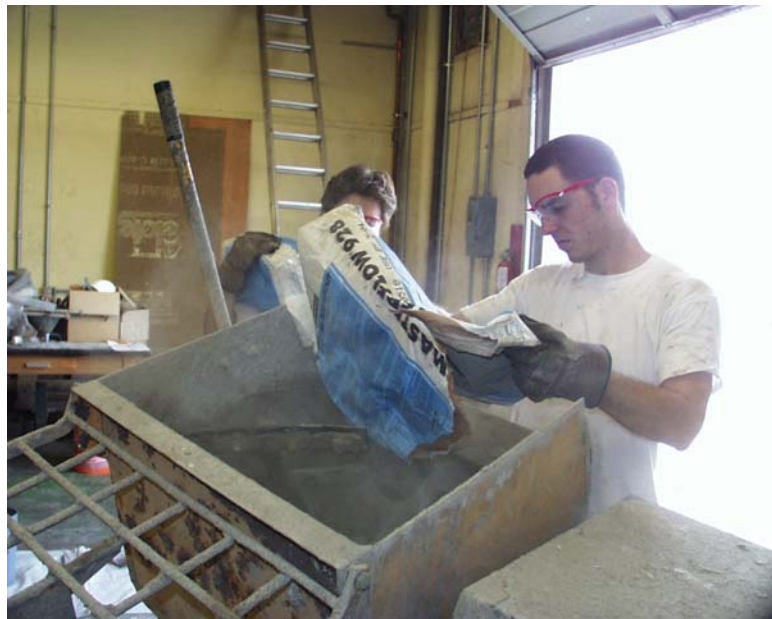
Figure C.3 Emptying of Grout Bags for Mixing
