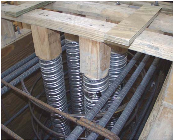
Figure 3.15 Vertical Alignment of Ducts during Concrete Placement
