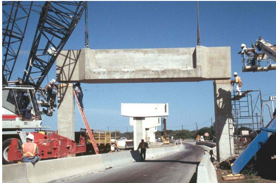
Figure 1.4 US 290 Ramp E-3 Project Precast Bent Cap
