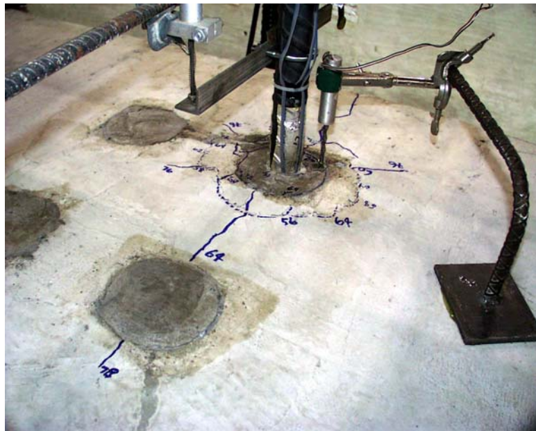
Figure 5.11 Splitting Cracks in Test No. 9
