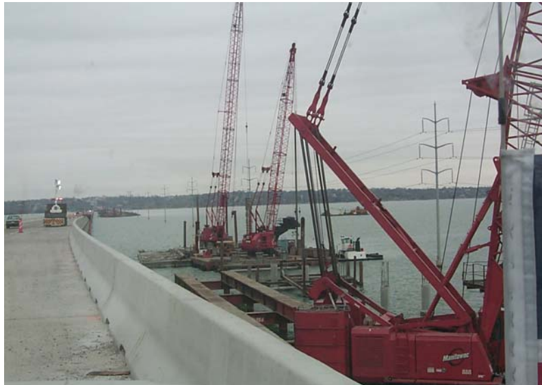
Figure 2.6 Lake Ray Hubbard Bridge Construction Site [2.8]
