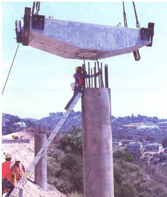
Figure 1.19 Precast Crossheads Used in the Getty Center People-Mover System Project [1.19]
